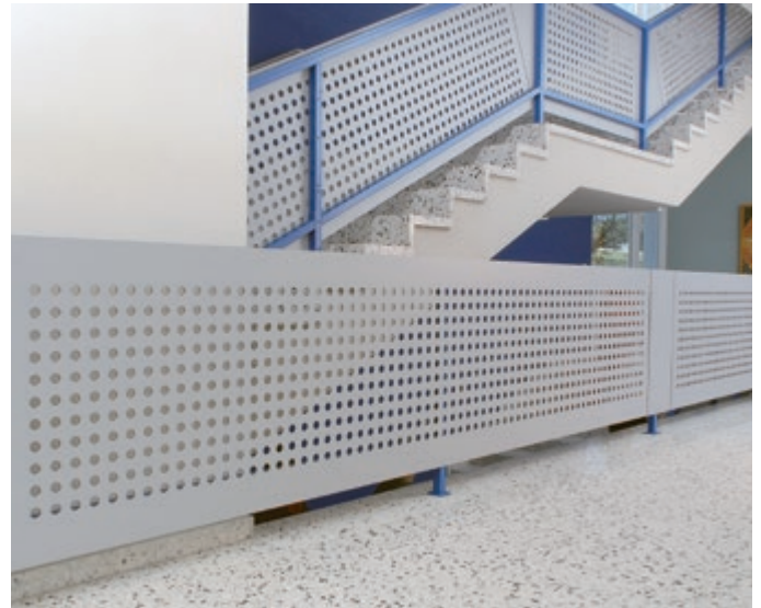
STAIR RAILING - HOLE MILLING
