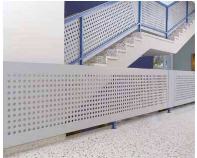
STAIR RAILING - HOLE MILLING
