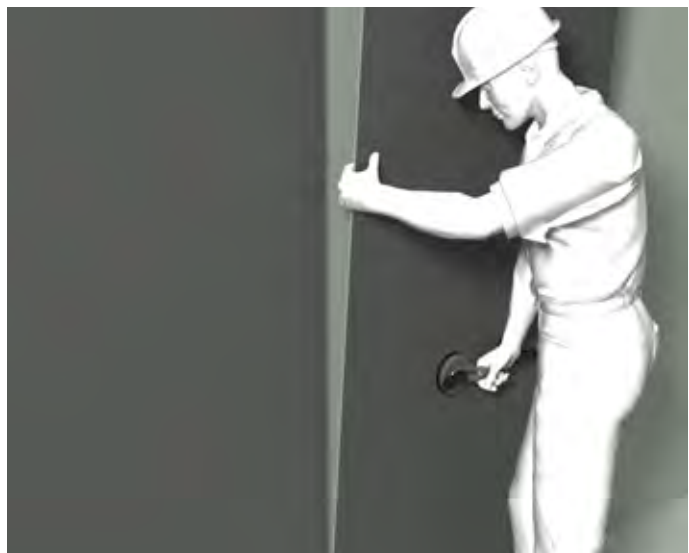
Place panels with suction handles
