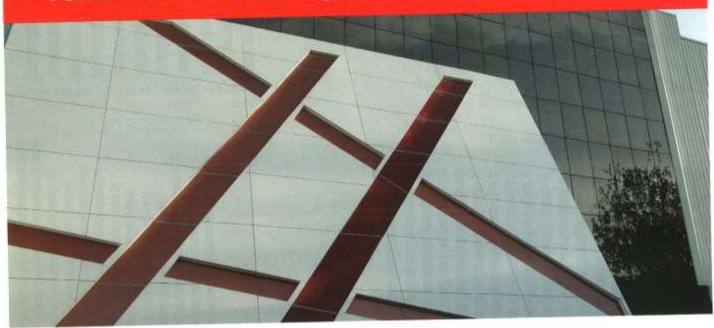
FunderMax's rear ventilated facades potentially improve buildings protection against noise pollution from outside. However, in this system the air cavity is almost totally open, fully ventilated and not very wide.
